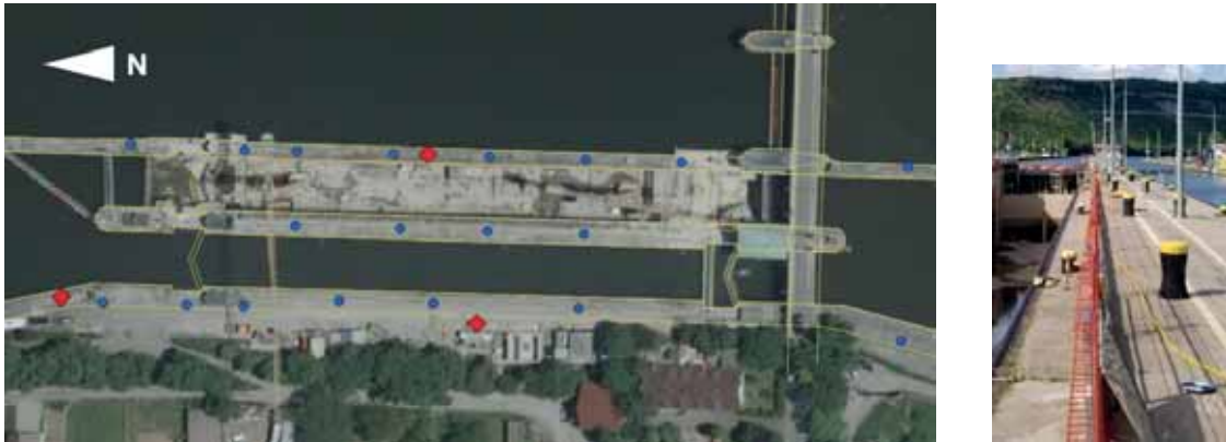
Fig. 3: Test area of ship lock Hessigheim/Neckar with distribution of signalized points. The image on the right shows one of the signalized points. All points are fixed to the ground except three, which are mounted on top of approximately 140 cm high concrete pillars (red squares).
