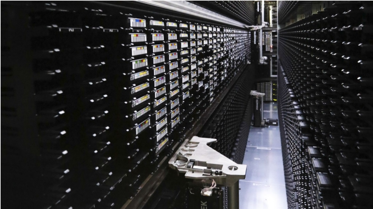
Fig. 3: DLR's StorageTek SL 8500 Robotic Tape Library
